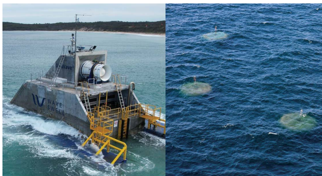
Fig. 1. Notable Australian deployments: Wave Swell Energy Uni-Wave 200 (left); Carnegie Clean Energy CETO 5 array (right).
